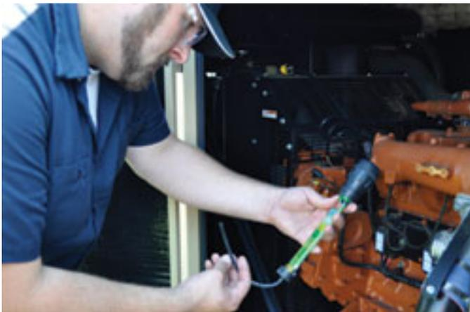
**The coolant thermal-protection level should be checked every six months. The general inspection**
