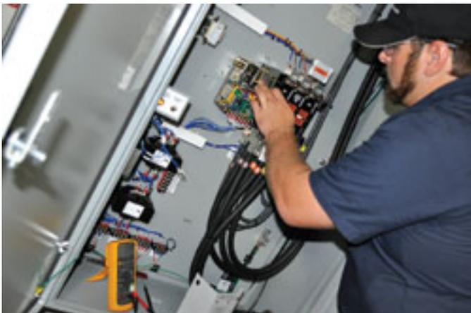
**Alternators require an annual inspection, as well as occasional testing of winding resistance.** OEMs provide detailed maintenance guidelines that should be followed to provide the longest most reliable service life possible for their respective equipment. General guidelines for specific applications also can be found in several recognized standards. One such standard is the *NFPA 110, Standard for Emergency and Standby Power Systems (2010)*
