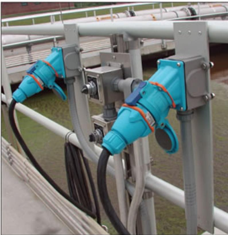
This close-up shows Meltric Decontactors for two different mixers. Pressing the pawl on top of each device safely disconnects the power before the plug and receptacle can be separated.
