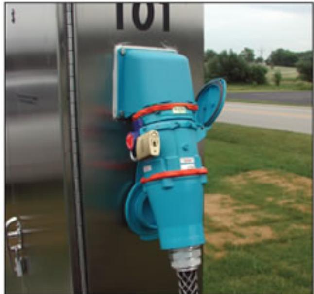
Unlike pin and sleeve devices, the Decontactor can be padlocked easily in the on or off position to eliminate the dangers of tampering.
